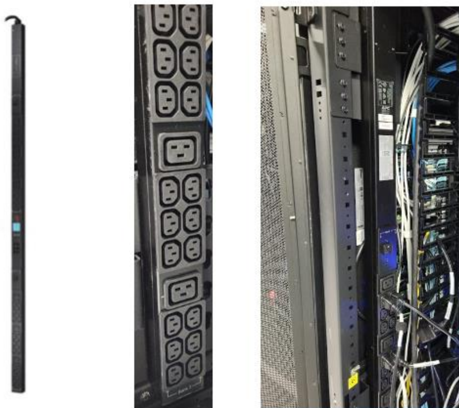
Figure 26: Smart PDU.
